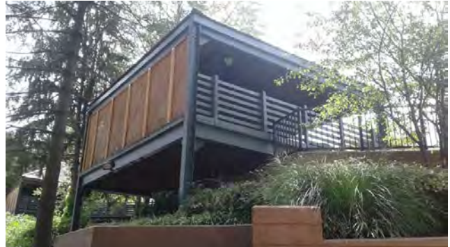
The installation of pavers and landscaping enhancements surrounding the gazebo.
