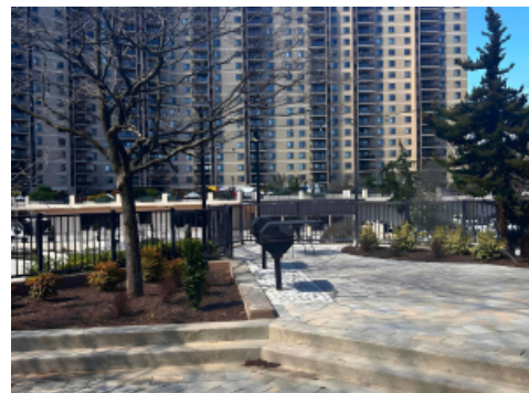
BrightView and Management transformed the Gazebo Landscape and Pavement area. Photo by: Brianna Hawkins.
